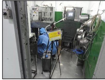
4. Factory 2 : Mixing Room 1
